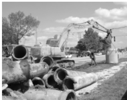
Workmen replace storm sewer pipes while widening Maple Avenue.
