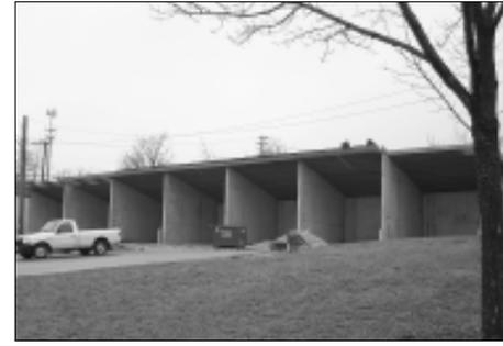
the local drainage system. Storing stone in a roofed structure eliminates this source of pollution.
