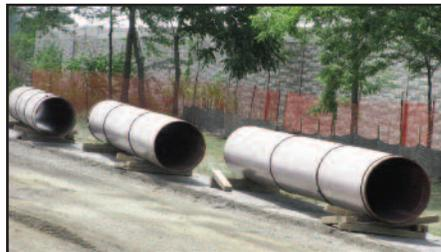
***BIG pipes staged for installation. NICOR is replacing their gas transmission line in their I-88 right-of-way. The Lisle portion should finish by September. The r-o-w will be restored with grass seed.***
