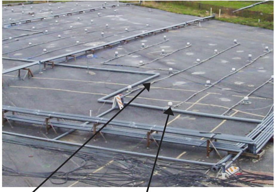
*These cables have been removed and these white electrodes will be cut off two feet below the surface and filled with grout as the electric heating cleanup system is phased out. The gray piping used to clean hazardous soil vapor will remain.*
